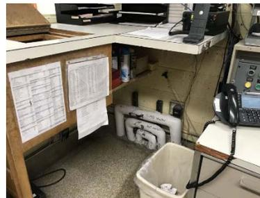
to communicate with the inmates. Some of the surrounding cabinetry is missing doors and drawer covers. Data lines are bound together, but left exposed and hanging on runs behind equipment. Chemicals were observed unlabeled and uncontrolled on top of electronic equipment. The overall appearance of the control room is cluttered and disheveled.
