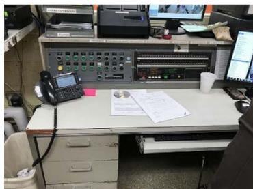
The equipment of the main control room is antiquated. The control panel is a refurbished countertop from an old dispatch center. The door controls only open a small portion of the doors within the facility. The remaining controls activate two way speaker systems
